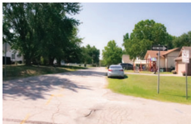
19th St looking south from 6th Grade Center with no sidewalks
