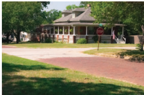
15th St & E 146th Street Intersection lacking sidewalk
