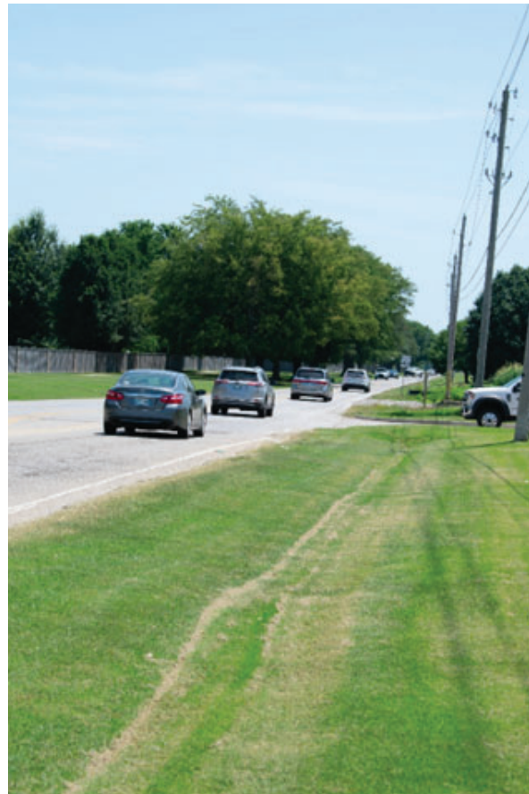
Mingo Road looking south from 101st Street with no sidewalk or shared use path and fully developed suburban neighborhoods on either side of street
